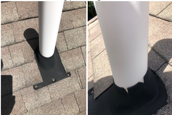
Cracked and curling plumbing vent boots:
